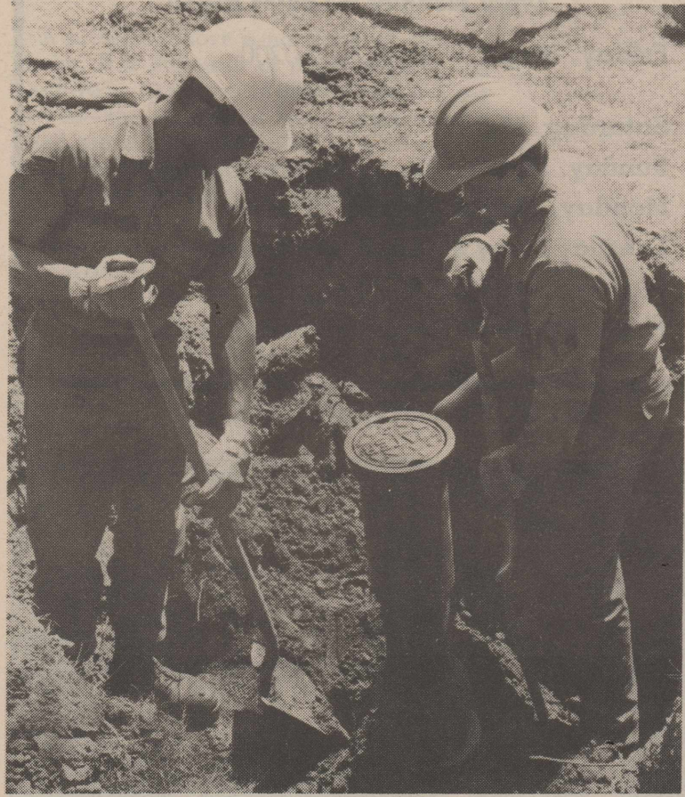
Sgt. T.B. Taylor (left) and A1C Mike Determan, 64th Civil Engineering Squadron Plumbing Shop, replace a 12 inch valve below ground for the Base Water Distribution System.
