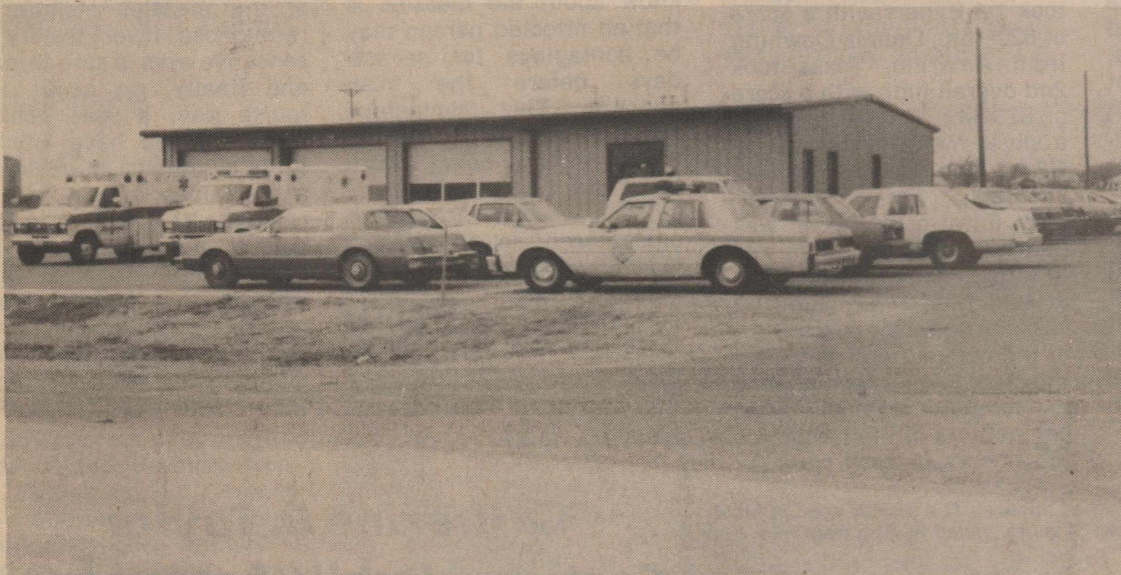
Coldwater Manor residents had to be evacuated into the Ambulance Building.
