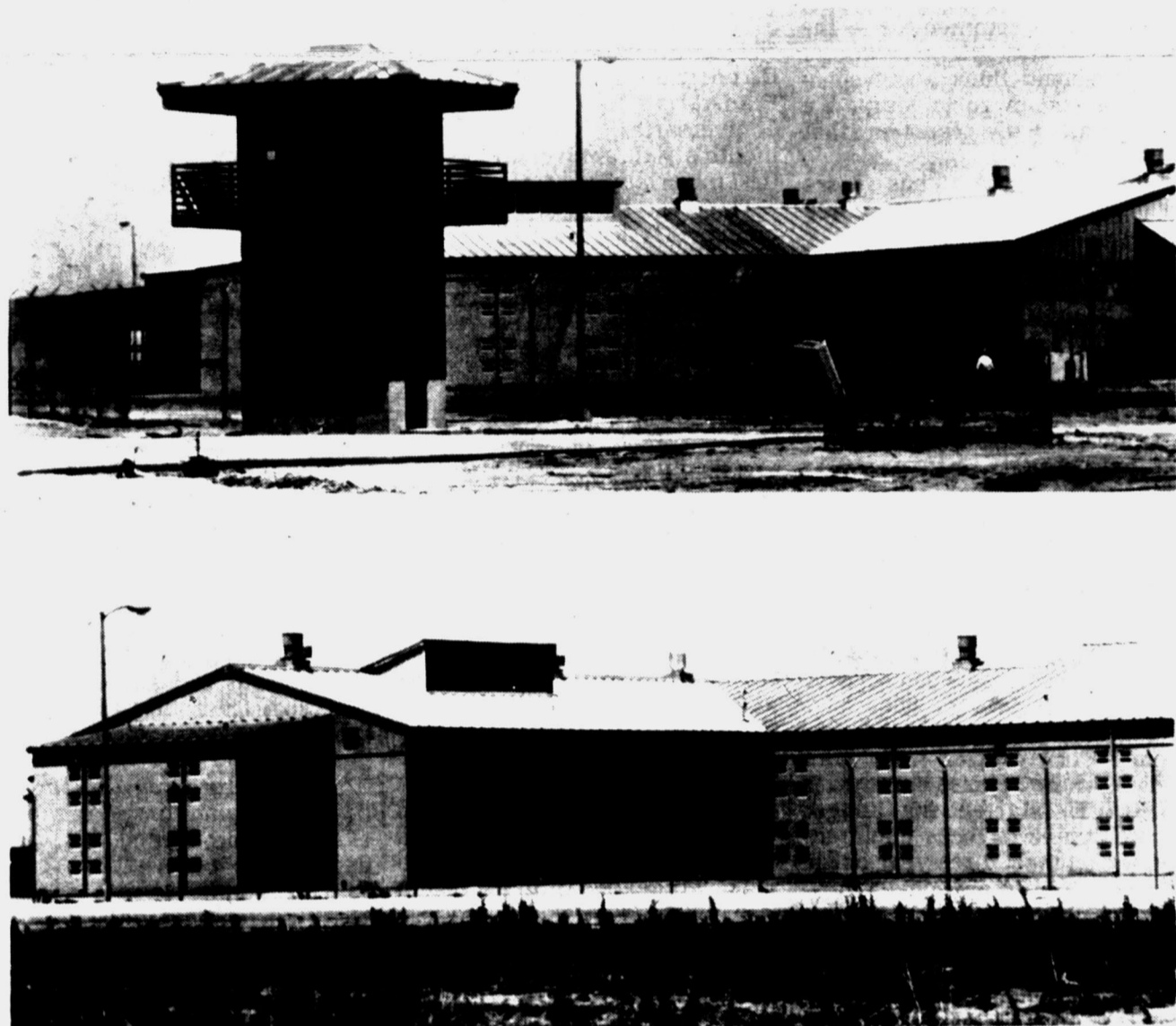
THE DANIEL UNIT — Snyder's new 1,000 man prison has taken shape and is nearing completion east of the city. A guard tower at the northwest corner of the unit stands in front of one of the four 250-man dormitories in the bottom left photograph, and one of the other dormitories is shown from the west side of the compound at top left. The
