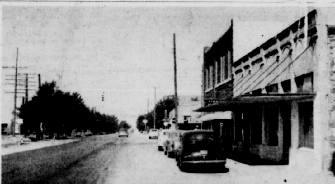
U. S. HIGHWAY 80 through Stanton as it appears today, looking west from downtown section. Business houses on right are built on the right-of-way line and the Texas and Pacific Railroad is adjacent to the south line of the 70-foot thoroughfare named North Front Street. 80-foot right-of-way needed for four lanes of traffic through the city may be secured by voters approval of a "land swap" with the railroad.—Reporter Staff Photo.
