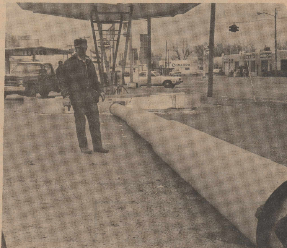
VICTIM OF WINDS-- The large EXXON sign which formerly stood just west of Bain Oil Company at the intersection of Highway 54 & 287 came down with a resounding crash last Thursday. Luckily, nobody was hurt and the end of the sign missed the gas pumps by only inches. Phillip Bain, station owner, said he had been afraid the sign had become loose and the winds of last week sent the huge sign crashing to the earth.
