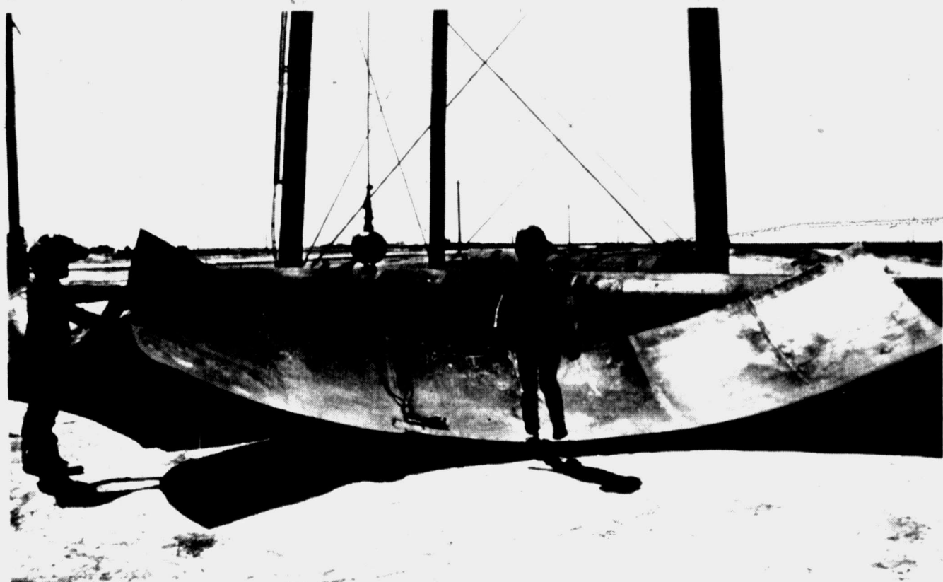
PUZZLE PIECES — Construction of the 150,000-gallon water tank at the prison site resembles putting together a giant puzzle. Here, worker Albert
