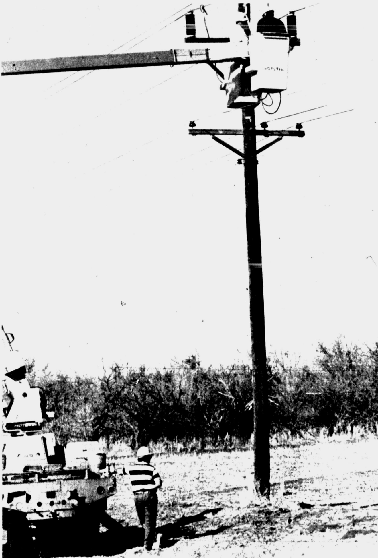
69,000 VOLTS — A TU Electric crew worked Wednesday afternoon alongside Ave. E north of Snyder to tap into a 69,000-volt line to supply Midwest Electric Co-op with the power to provide
