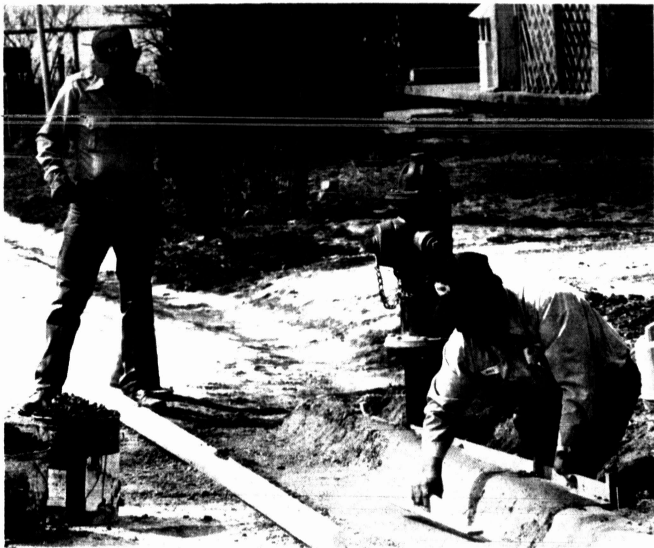
REPAIRS — Paul Gutierrez, right, and Tommy Guynes were repairing a gutter and fire hydrant on Ave. T near the county library Thursday. (SDN Staff Photo)
