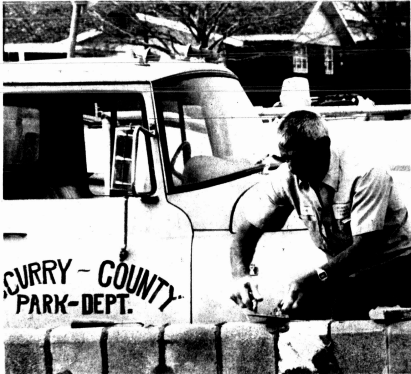
WORK AT PRAIRIE DOG TOWN — County park employee Bob Prozeller is pictured repairing cracks in the prairie dog town fence in Towle
