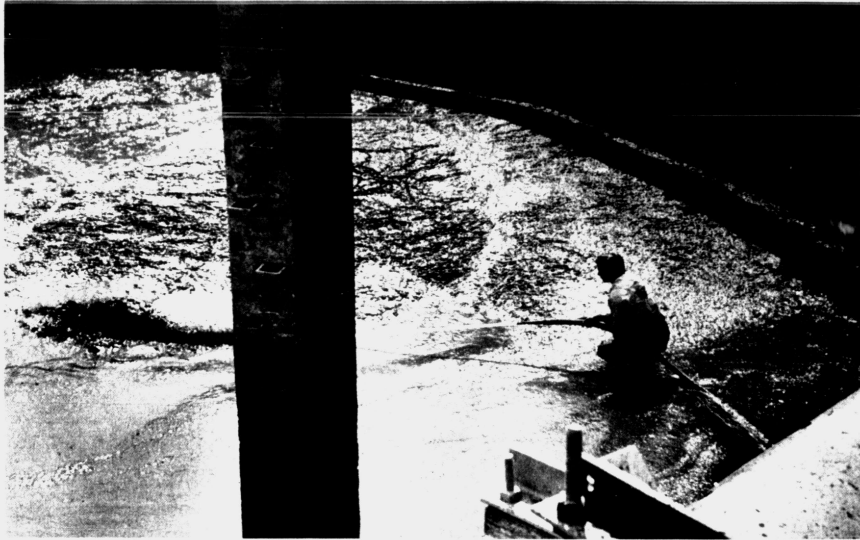
CLEAN UP — Shannon Warner is pictured using a fire hose to wash away mud in the "Sedimentation Basin" at the W.S. Bigham Water Treatment Plant. The basin requires periodic cleaning in which plant workers must shut off water to the plant, drain the basin and
