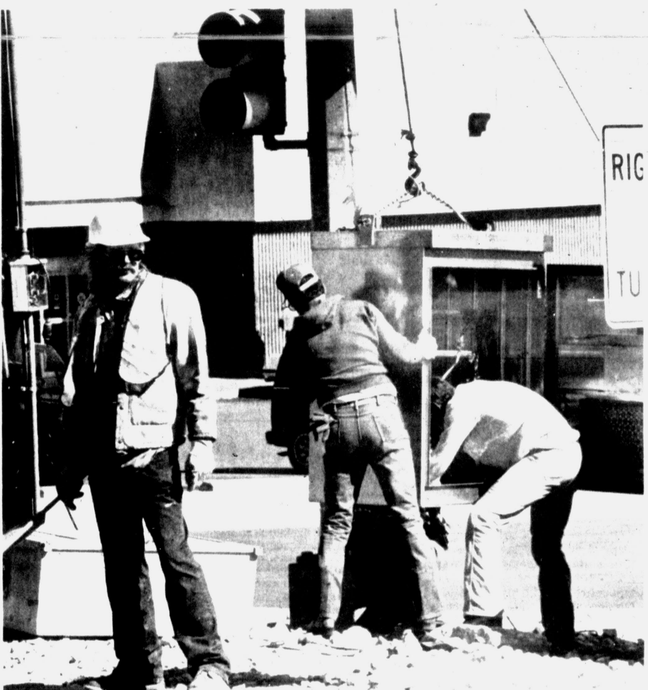
FAST FIX — Paul Lawson, left, Sonny Thompson and Bill Rister of the state highway department were moving quickly to fix the stoplight at 30th St. and College Ave. during the noon hour Wednesday. (SDN Staff Photo)
