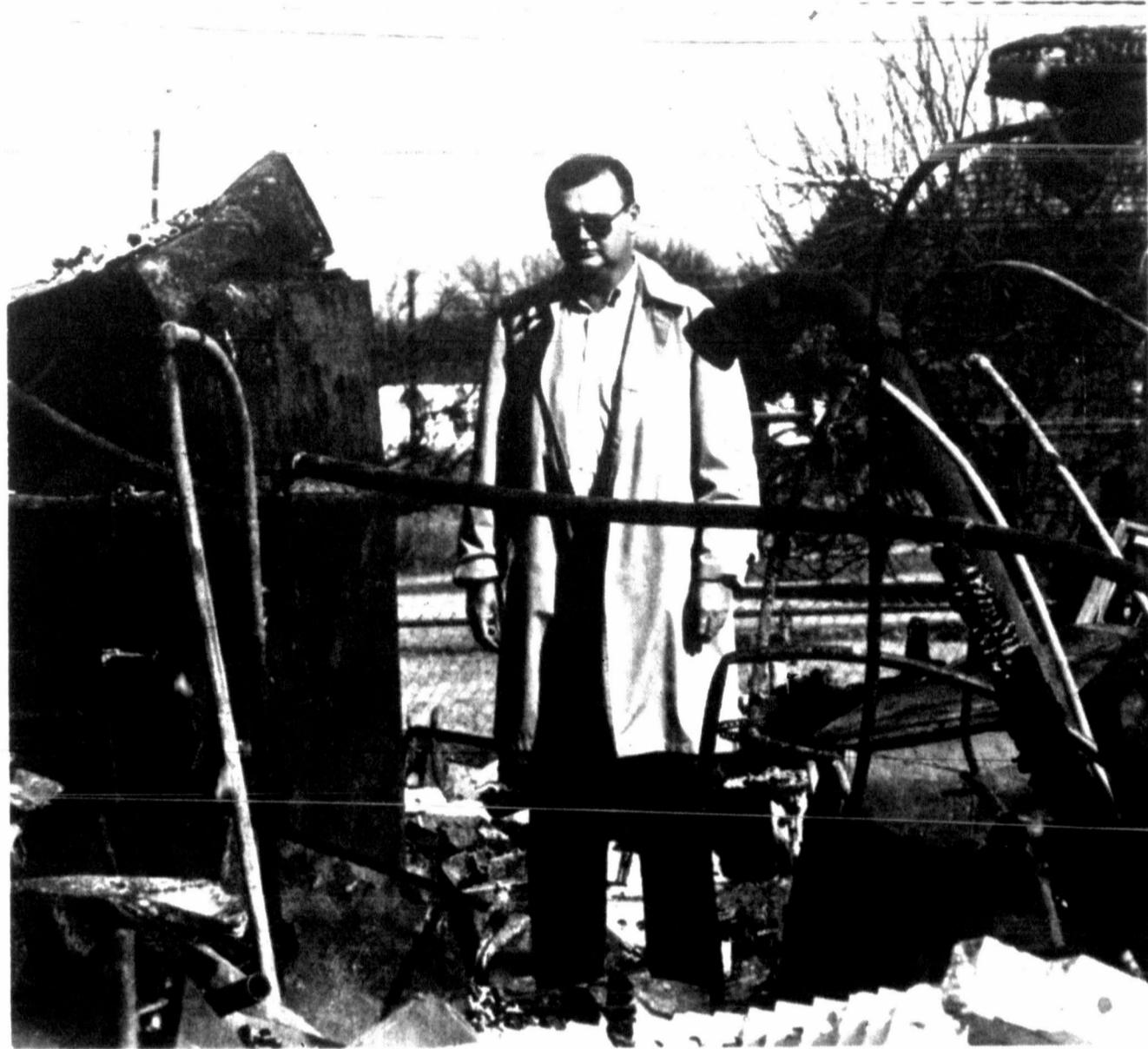
AFTERMATH — Fire Chief Terry Don McDowell inspects the rubble that was the Ave. D Baptist Church sanctuary building. The church fire was one of several recent major fires here that happened in extremely cold weather. (SDN Staff Photo)
