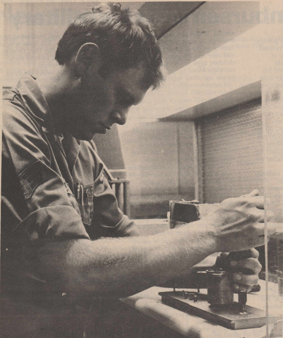
SrA Gary Hansen disassembles a gearbox coupling from a J-85 T-38 engine. He has been assigned to Reese AFB for three and one-half years. He is a machinist assigned to the Fabrication Branch of the 64th Field Maintenance Squadron.
