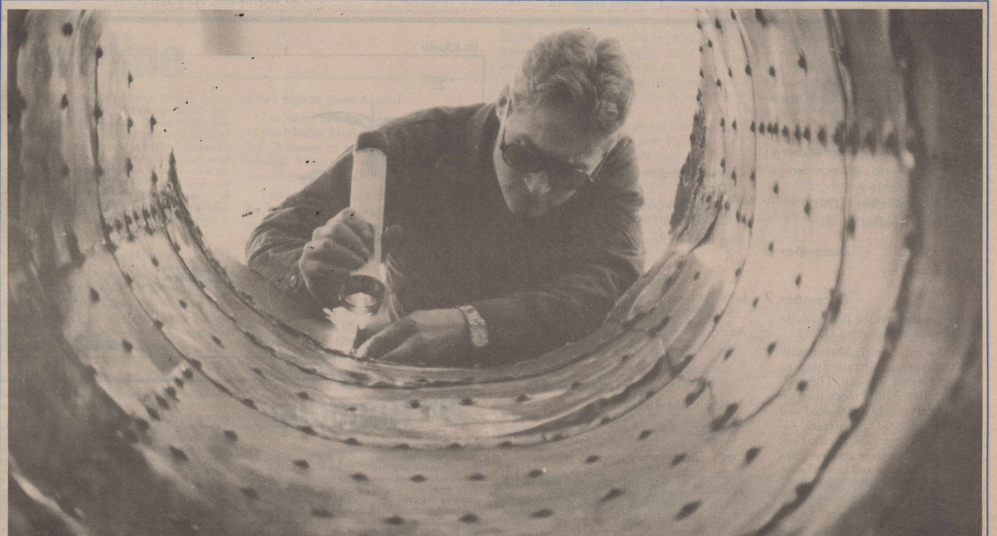
SrA. Gerald Carrell, a dock mechanic assigned to the 64th Organizational Maintenance Squadron checks for foreign objects in a T-38 boattail. SrA. Car-
