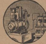
Delco-Light has already proven satisfactory in the telephone industry for country towns. For a common battery exchange, Delco-Light will charge the storage battery for both ringing and talking. It will furnish electric light for all parts of the
