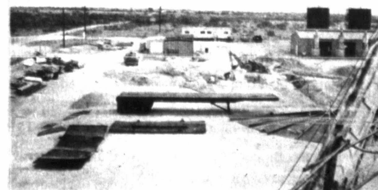
WATERFLOOD PROJECT — Exxon's East Vealmoor field secondary recovery project is on schedule. Photos show new salt water storage tanks, an operations control building and crews burying electrical conduit. An identical project begins this month in the Sharon Ridge field. (Exxon Photos)
