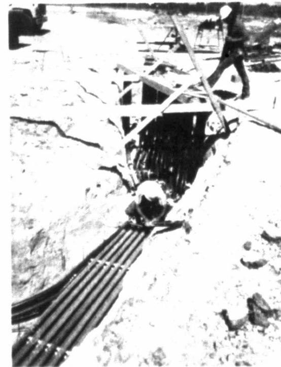
WATERFLOOD PROJECT — Exxon's East Vealmoor field secondary recovery project is on schedule. Photos show new salt water storage tanks, an operations control building and crews burying electrical conduit. An identical project begins this month in the Sharon Ridge field. (Exxon Photos)
