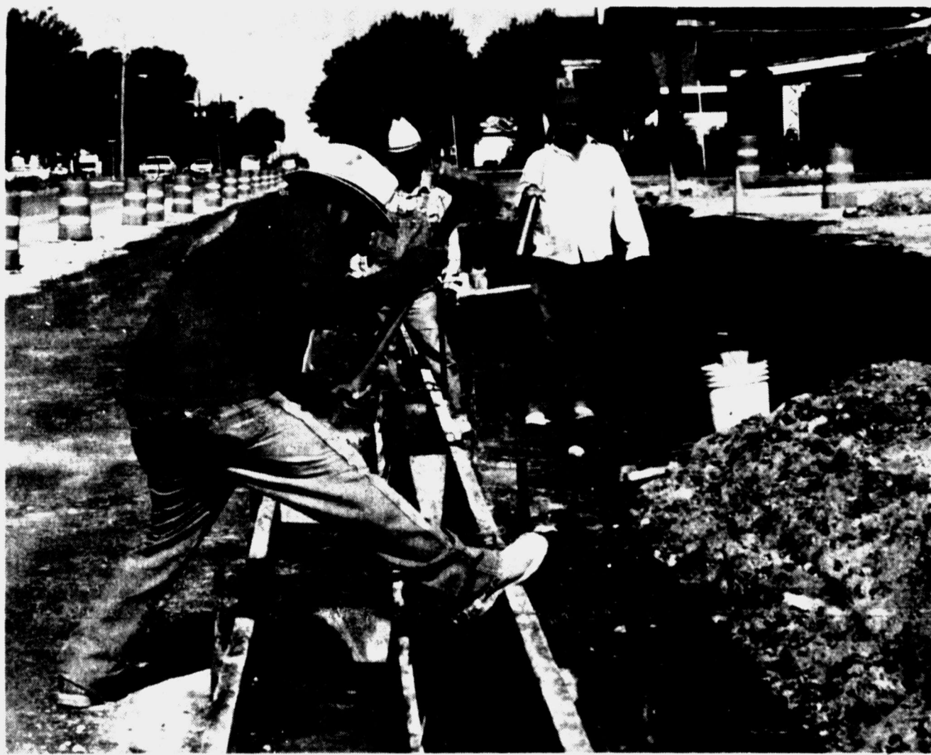
37TH STREET WORK CONTINUES — Crew members from Ortiz Construction of Lubbock prepare to pour more curb work this morning as the widening project along 37th St. continues. Curb work along the north side of the street is expected to be completed in the next couple of weeks. (SDN Staff Photo)
