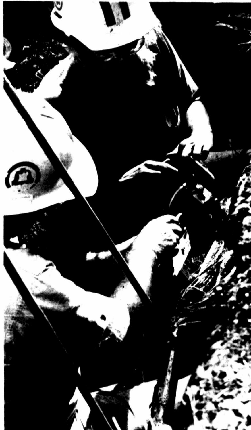
TEDIOUS WORK — Rick Wood and Debbie Allford match some of the 900 pairs of damaged phone lines which were accidentally cut when Southwestern Bell crews worked to put in additional anchors for utility poles across from the police station. Communications were out for about four hours Thursday and involved the police and fire stations, City Hall and a number of businesses and residences. (SDN Staff Photo)
