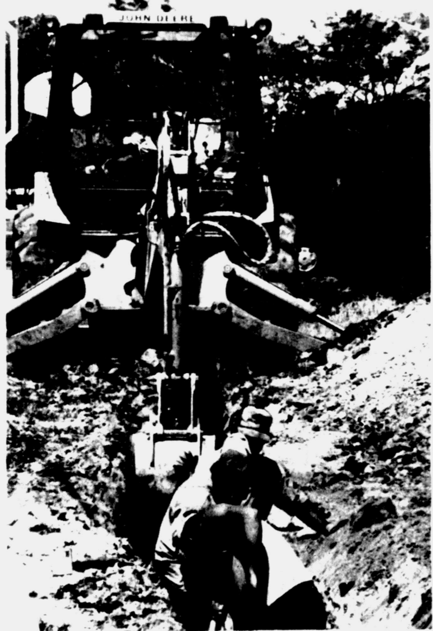
MORE 37TH STREET WORK — City crews have been assisting TU Electric in burying electrical lines along 37th St. The City crew is installing plastic pipe and will allow TU crews to install the wiring. Pictured are Darryl Boone, William Myers, John Flores and Juan Becerra. (SDN Staff Photo).
