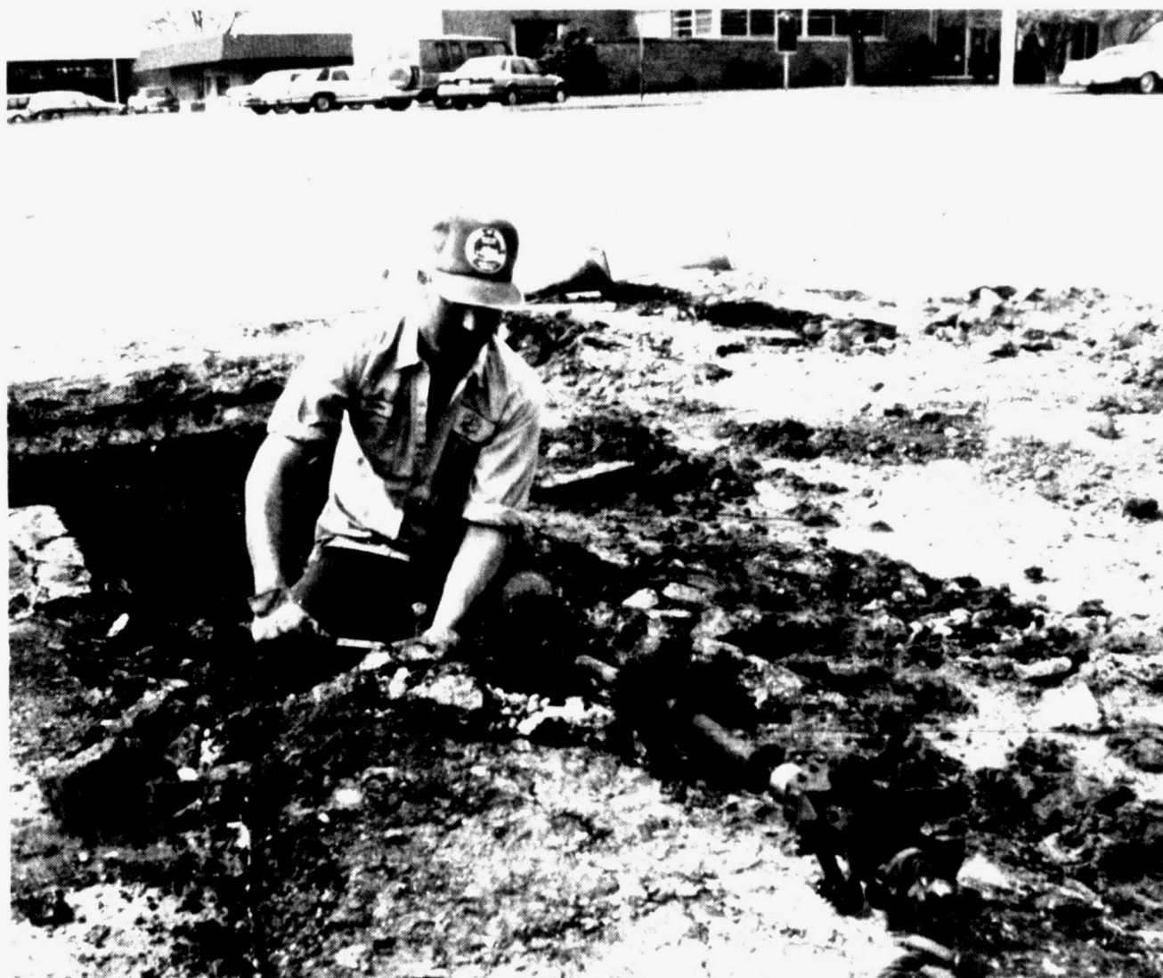
CLEANING THE LINE — City employee Alvin Dodson attaches this "brush" to a cable that will be pulled through city water lines to clean them before a cement lining is added. The process is part of the city's water line rehabilitation project along Ave. T. (SDN Staff Photo)
