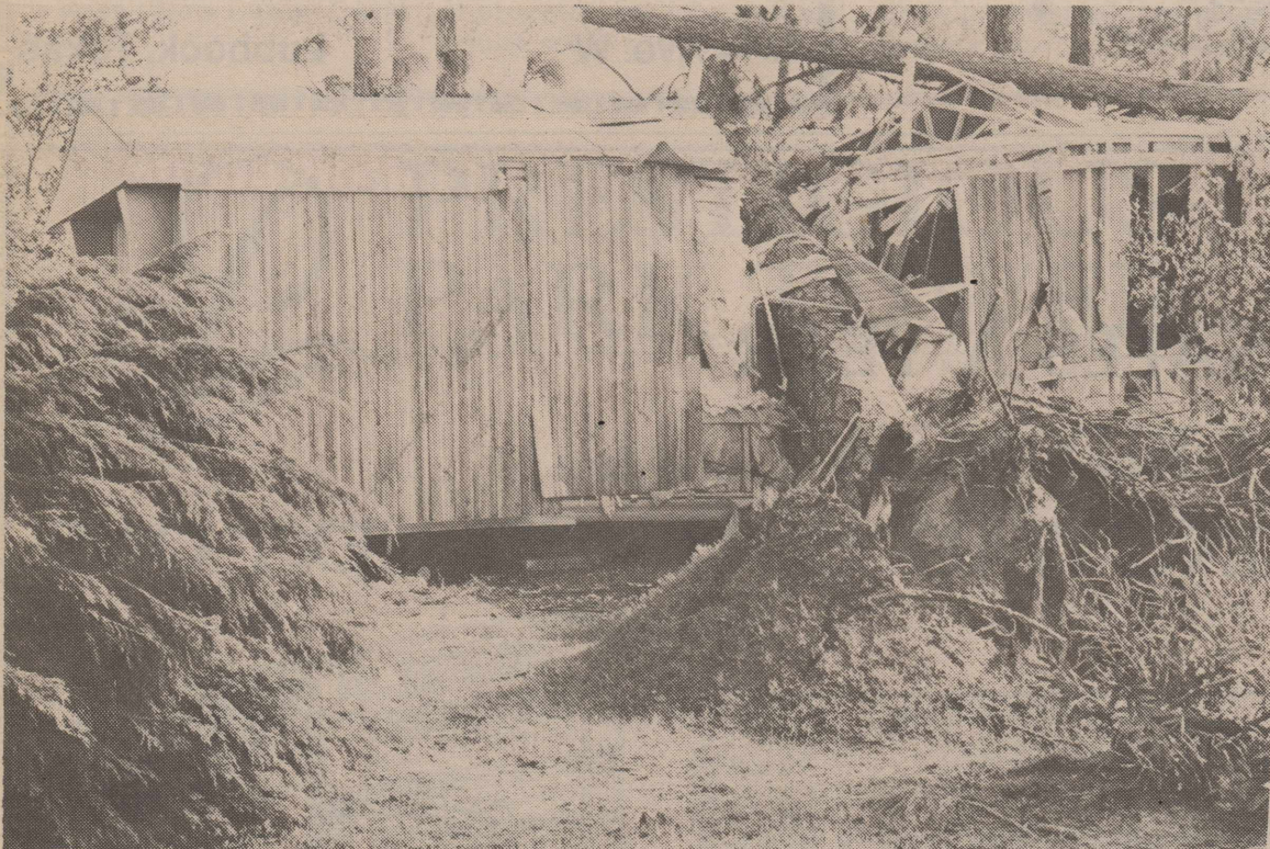
Hurricane Elena's high winds uprooted this tree sending it crashing into this building near Pascagoula, Miss., about 70 miles east of Keesler AFB.
