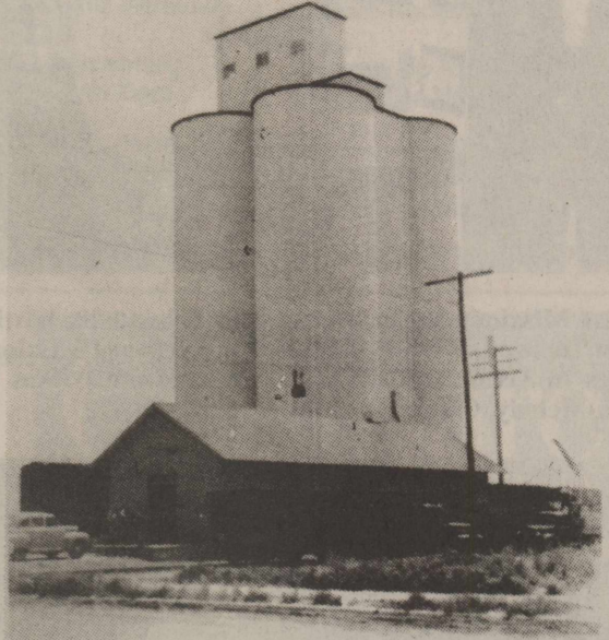
The new 125,000 bushel elevator completed at Stratford in February by Riffe Brothers.
