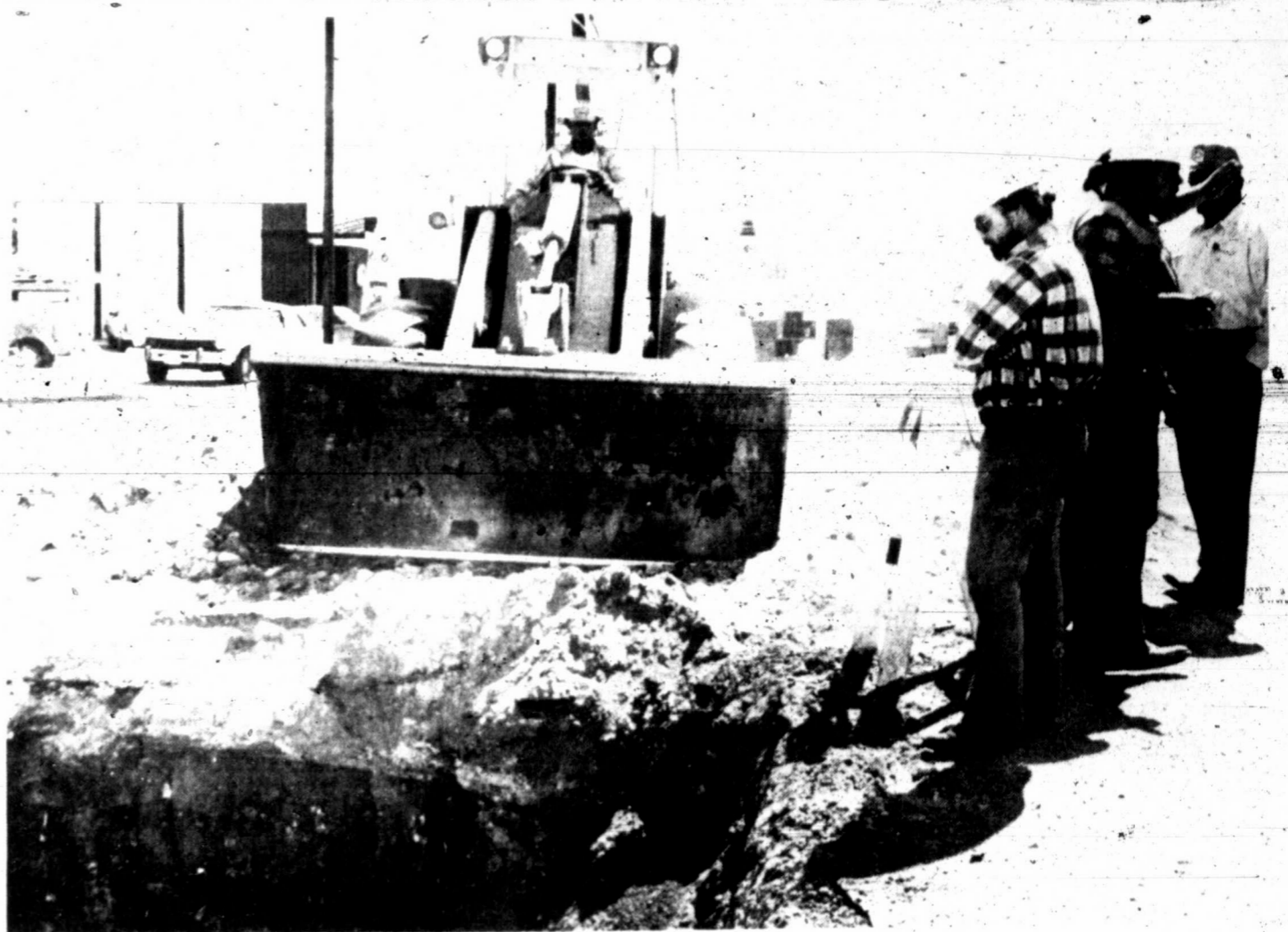
CABLE WORK - Work is continuing in the laying of underground conduits for Southwestern Bell Telephone. The work started several months ago and is expected to be completed by about Christmas. The photo above was taken at the intersection of 37th St. and College Ave. where telephone workers and contractors were preparing to install a manhole. The work covers the length of North College Ave. (SDN Staff Photo)
