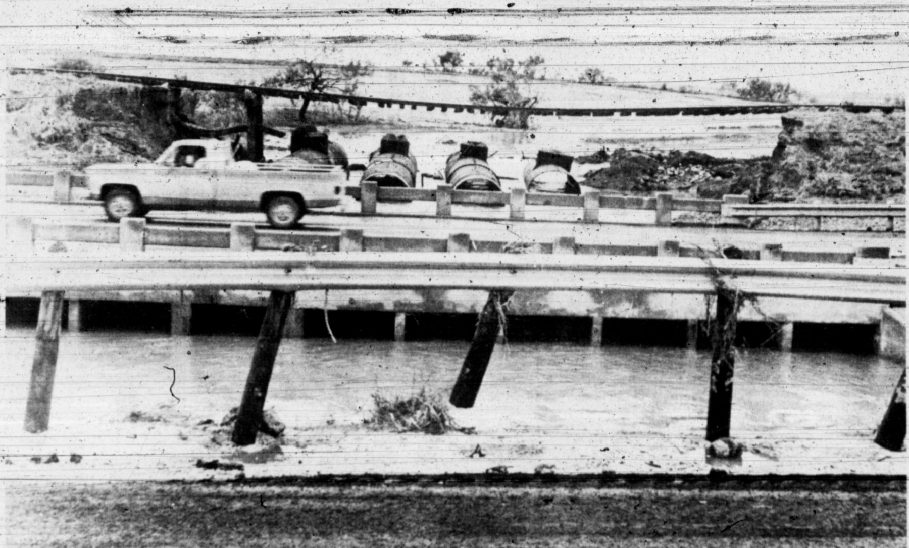
WEATHER SCENE -This railroad bridge (background) about 24 miles southeast of Snyder on U.S. Highway 84, couldn't handle the amount of water that wanted to go under it Tuesday and as a result, the bridge went downstream leaving only the tracks to span the chasm. A guardrail was about to follow when the water finally subsided. Roland Langford, who farms in the area, reportedly lost several head of cattle to the rushing water. (SDN Staff Photo)
