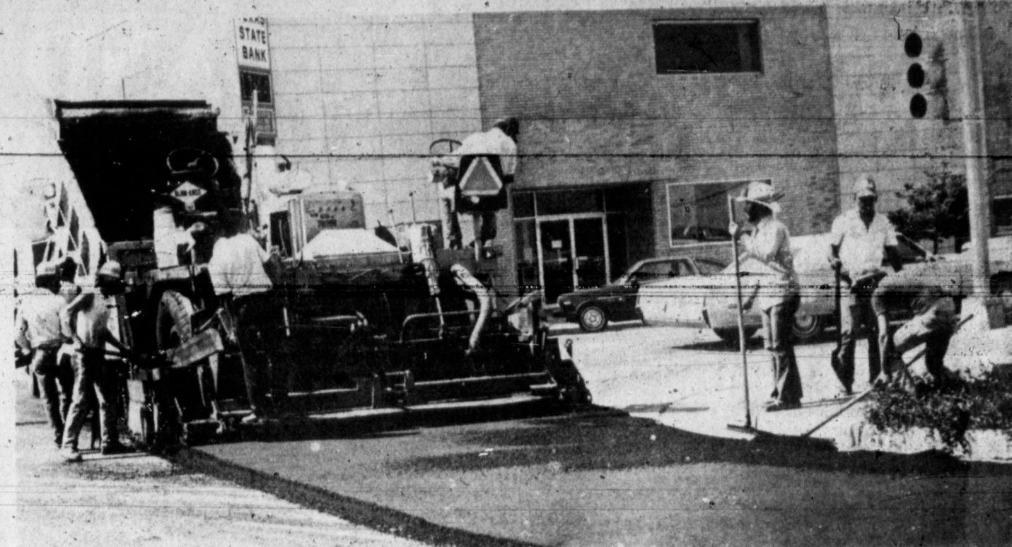
SMOOTHING IT OUT -Streets maintained by the state in Snyder's central business district are getting a new coat of paving material this week. The asphalt overlay of brick pavement, which has been in use for
