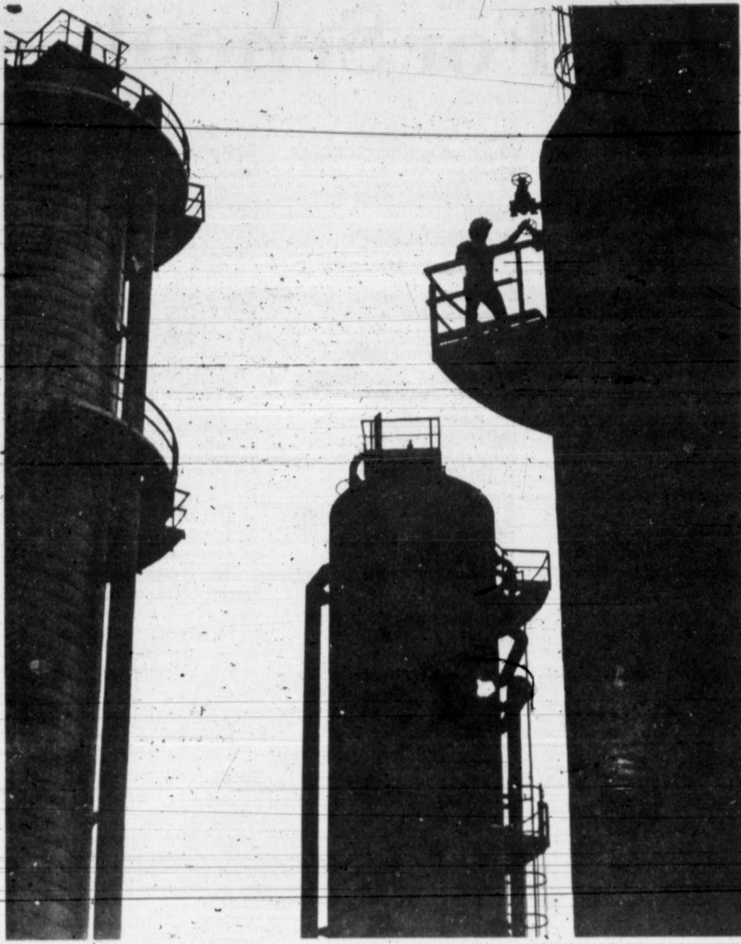
LOFTY PERCH —Amid the tall towers at Tenneco Inc.'s Petro-Tex chemical plant in Houston, Assistant Stillman Tommy Drouillard appears small indeed as he operates a valve from this lofty perch. Petro-Tex is a leading producer of MTBE, a blending agent that increases the octane rating of unleaded gasoline.
