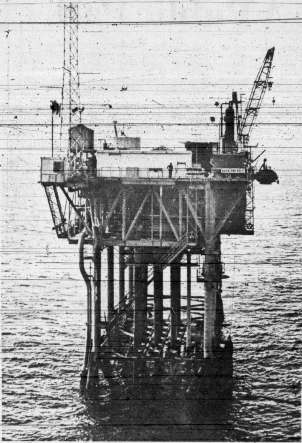
TAPPING THE GULF—Offshore platforms in the Gulf of Mexico tap into underground reservoirs of natural gas. Some of the gas produced at this platform, operated by Aminoil USA, Inc., supplies Texas homeowners with fuel for cooking and heating. Moving constantly through transmission pipelines, a cubic foot of gas would reach Texas about 17 hours after leaving this platform 250 miles away.
