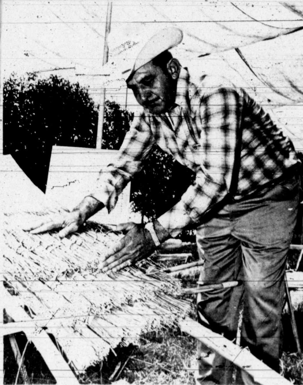
AT FOLK FESTIVAL—Juan E. Martinez of Laredo stacks bundles of grass to make a thatched roof. Other pioneer crafts such as shingle splitting, syrup making, chimney building and horsehair rope spinning will be demonstrated at the ninth annual Texas Folklife Festival, on the grounds of The University of Texas Institute of Texan Cultures at San Antonio, July 31-August 3.
