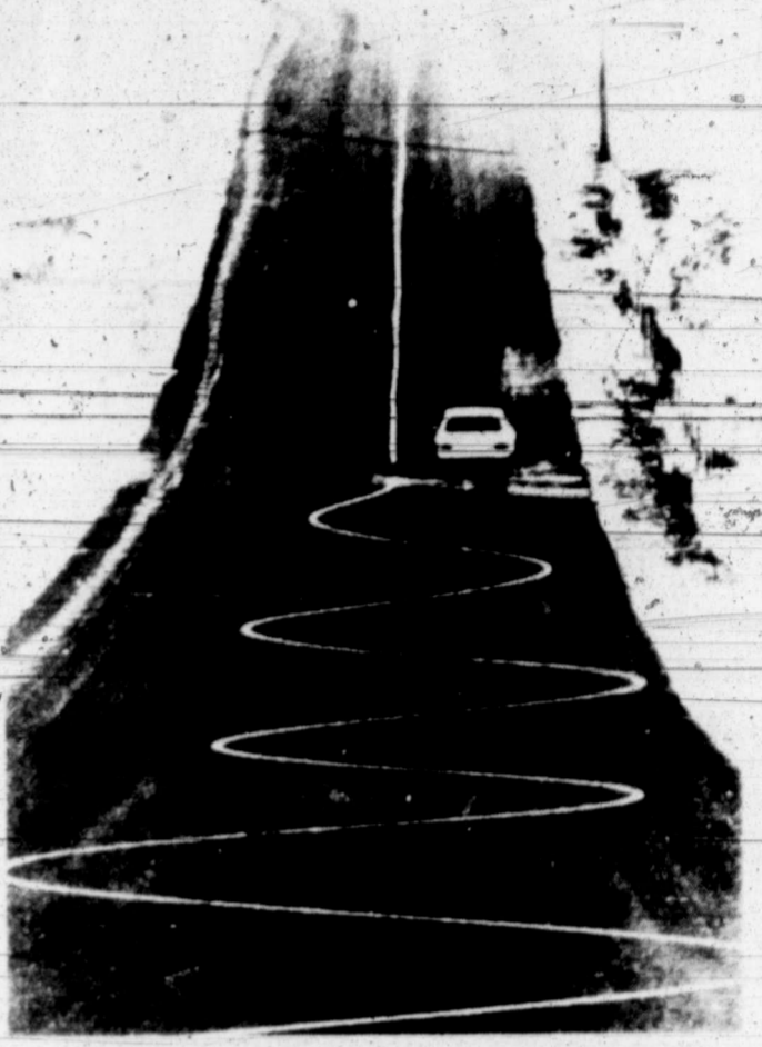
THERE IS A NEW twist to the line down the center of this road near the Sacramento, Calif., suburb of El Dorado Hills. The unusual line warns motorists that a dead end is just over the next rise.
