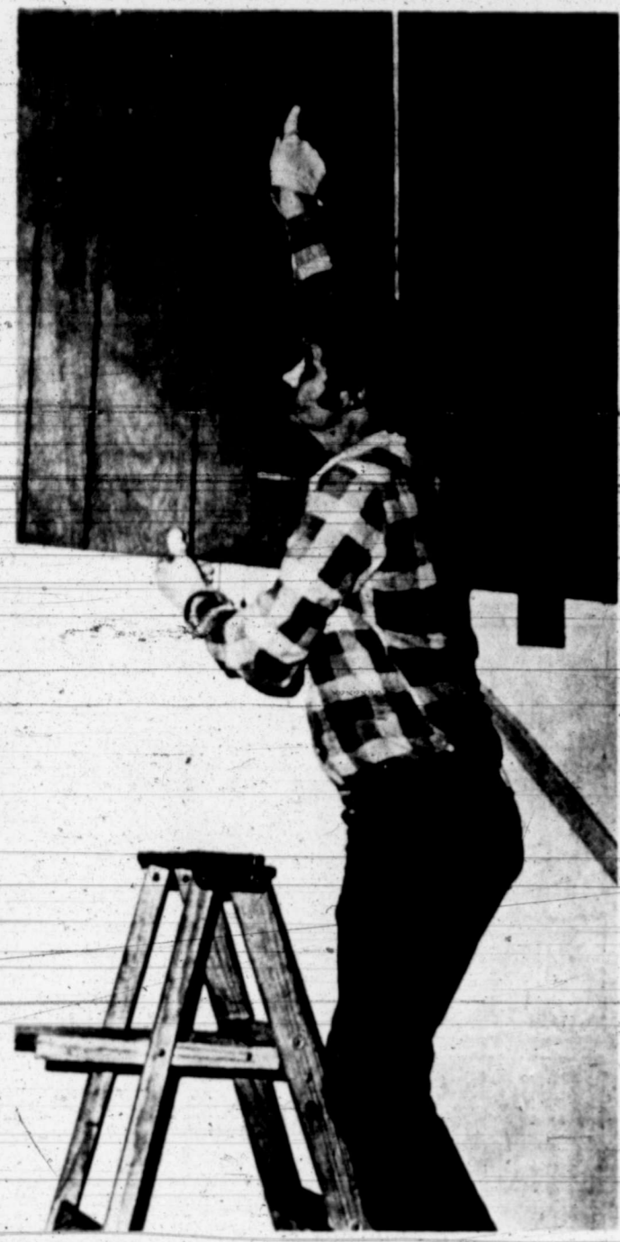
RENOVATING—Fenton's Dad & Lad, located on the east side of the square since 1952, will be moving into the old Top Dollar building on the north side of the square. Renovation work on the Top Dollar building has already started. Danny Fenton, above, removes some panelling. (SDN Staff Photo)
