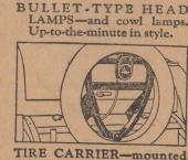
free from the body; rigidly supported by steel brackets
