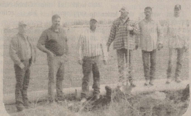
Ground breaking for the City's new Water Loop gets the project moving forward. Pictured above (l to r) Don Nicholson, City Administrator, Mayor David Brown, and Ricky Lawson, Project Superintendent and three Triple L employees
