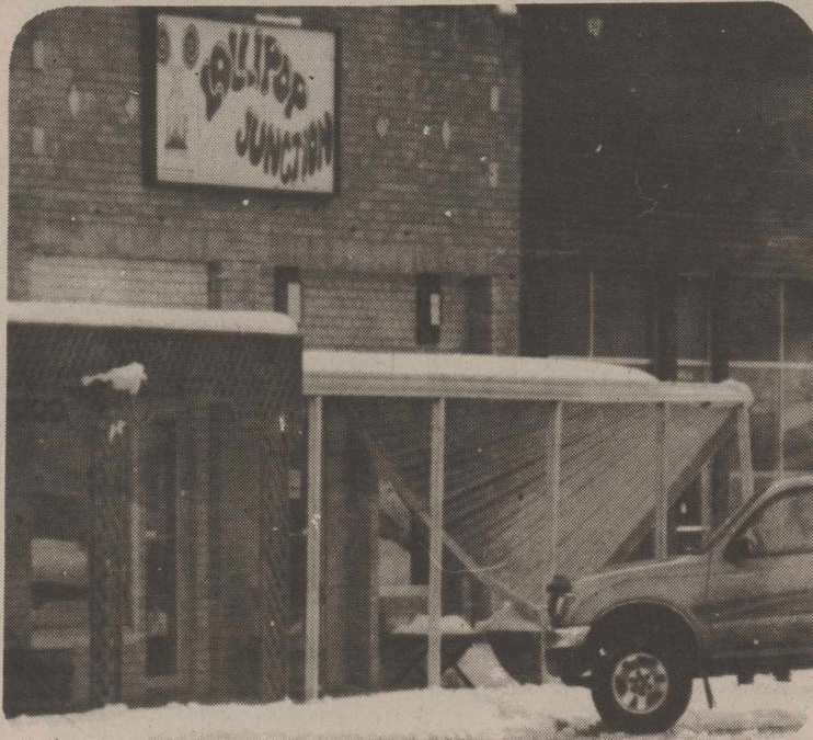
The awning at Lollipop Junction buckled under the weight of the snow over the weekend
