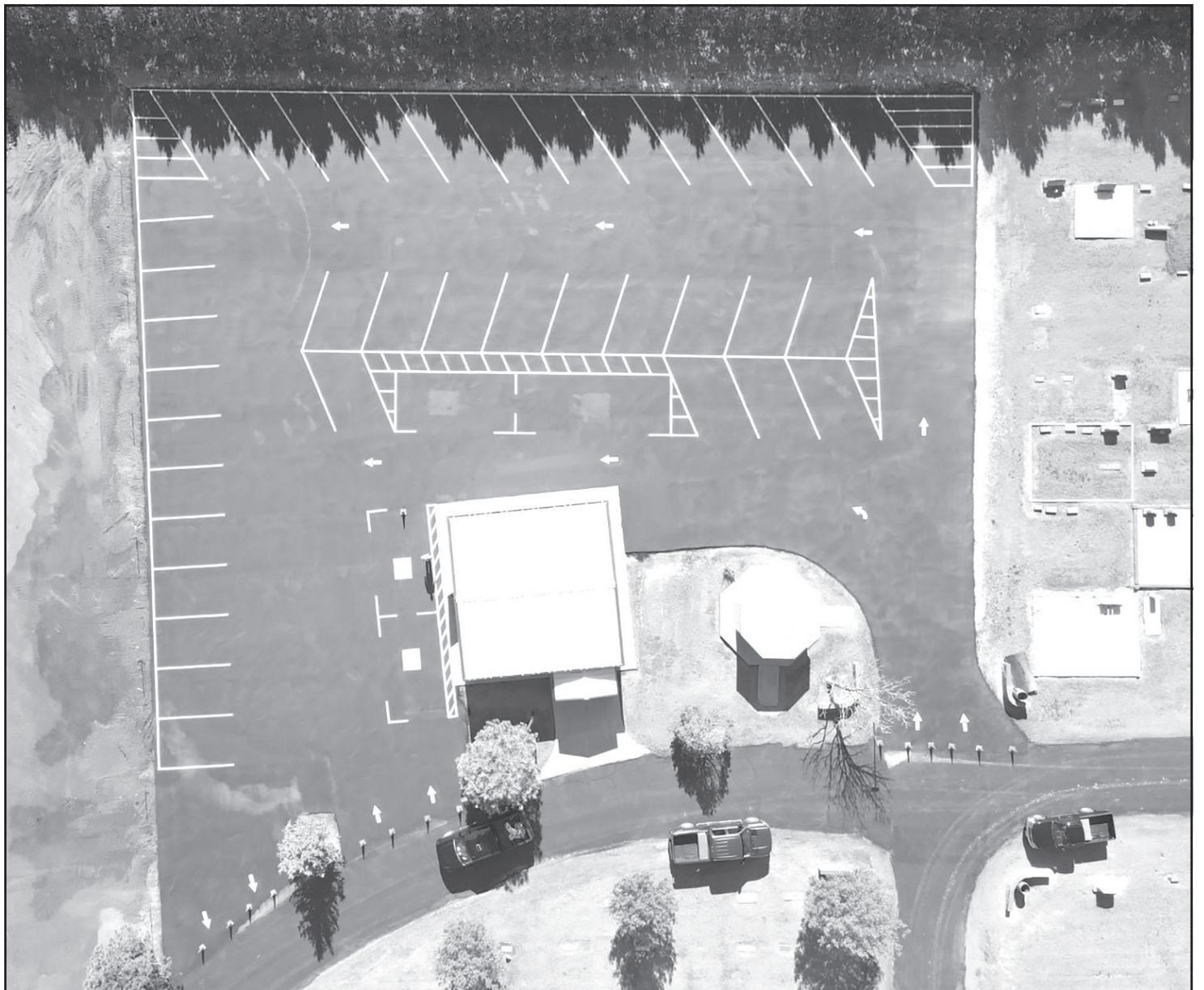
Richard Bermea sent in this photo, taken by a drone, of the new parking lot around the chapel at the Friona Cemetery. Cemetery "Clean Up" Day is scheduled for Thursday, May 20th. Work will begin at 5:00 p.m. at the Cemetery. There will be refreshments available in the Chapel. Everyone is invited to come out and see the new parking lot and help clean up our Cemetery.
