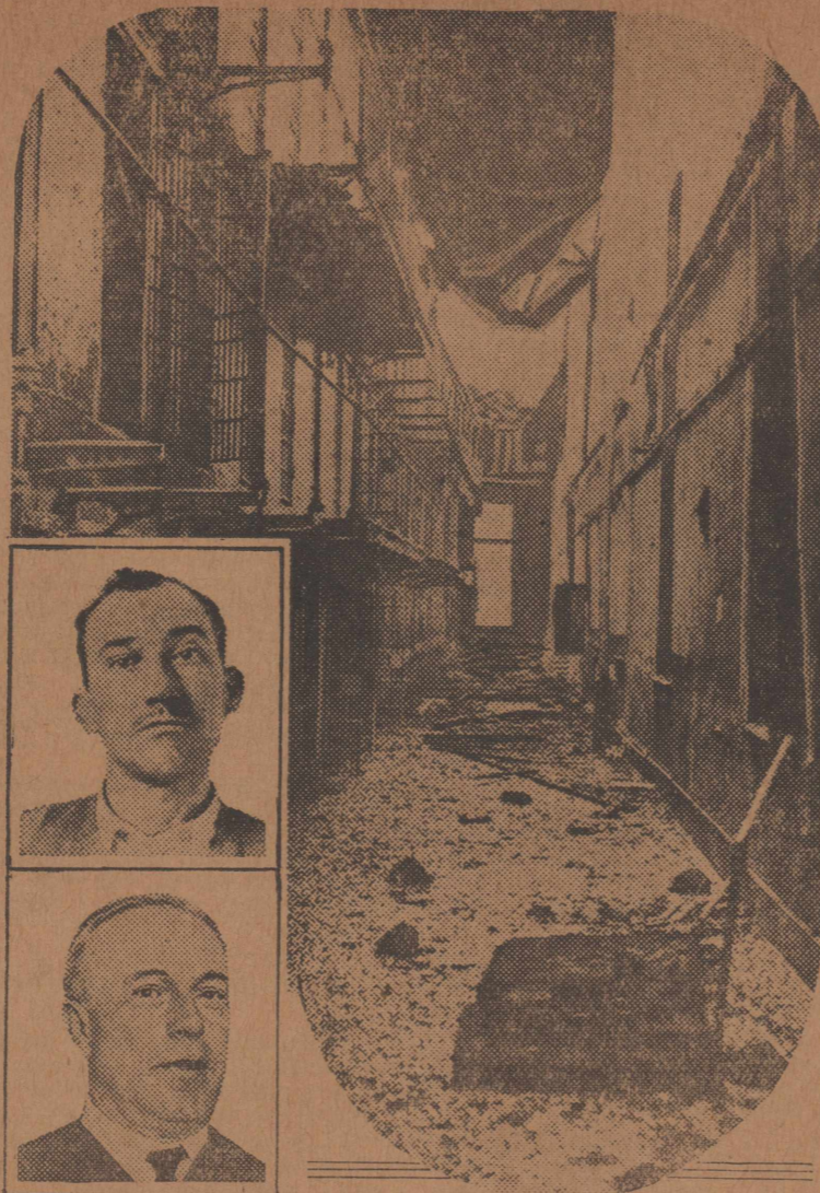
This shows the wrecked main corridor of cellhouse No. 3 at the Canon City, Colo., penitentiary which was used as a stronghold by prisoners, led by the desperado "Danny" Daniels, in their attempt to escape. It was in this cellhouse that seven guards were killed by Daniels and also here that Daniels, after efforts for freedom had proved futile, lined his ringleaders against the wall and shot them before killing himself. Daniels is shown in the top inset; the lower inset shows Warden Francis E. Crawford.
