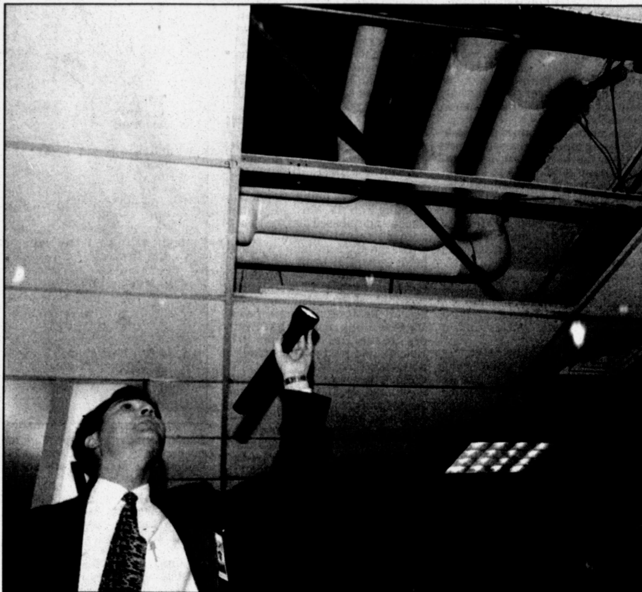
Ken Day points out that there is not enough room between the roof and the ceiling to add air conditioning and heating ducts that would be required to handle the present cooling and heating needs of the facility.
