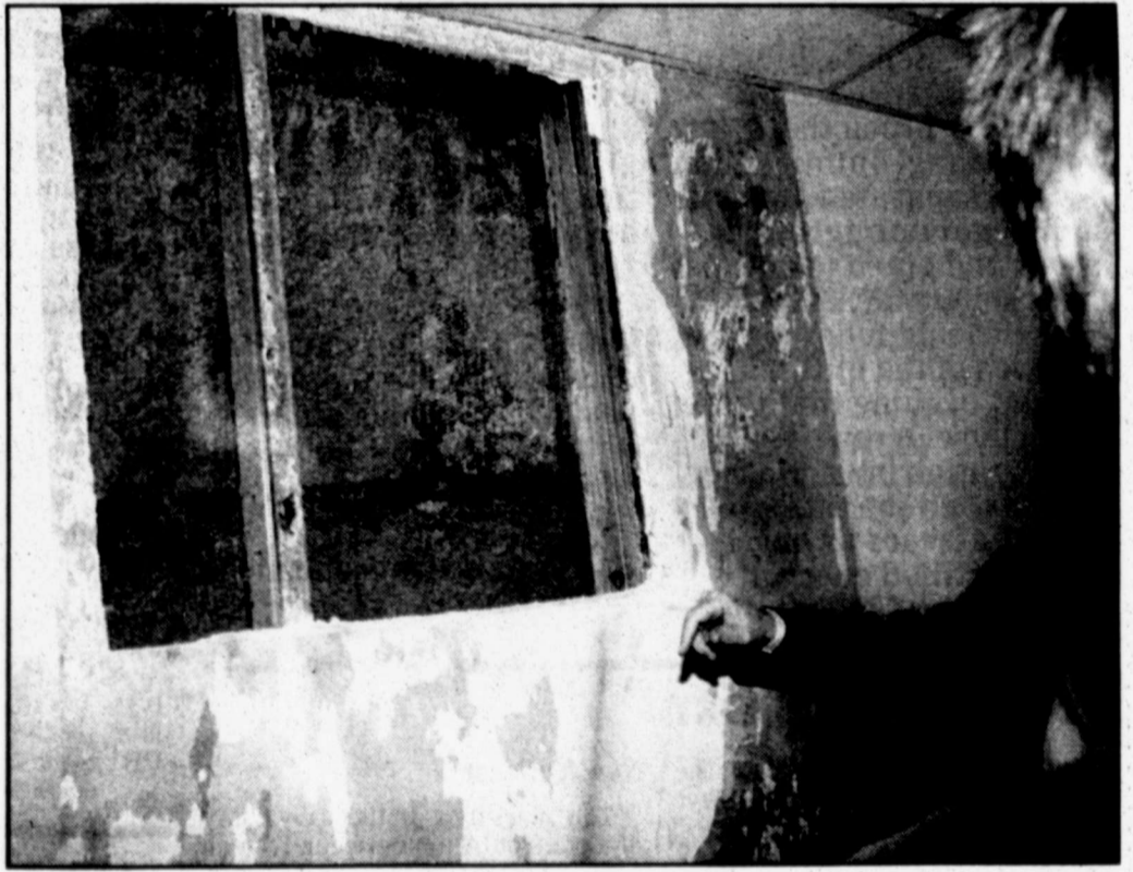
A section of the concourse shows how thin the walls are and adds to the problem of keeping the concourse cool in the summer and warm in the winter.
