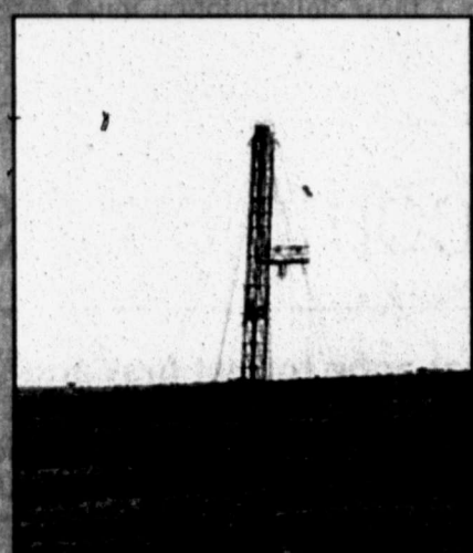
Open spaces surround a drilling rig.
