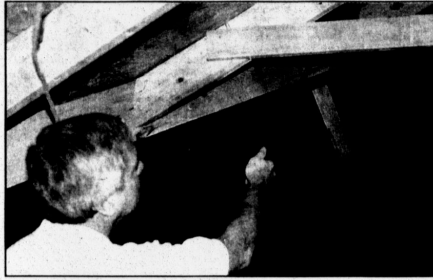
FireStop's Bill Wiley protects a family from fire danger by treating their attic with Nochar's Fire Preventer. Nochar is a non-toxic, environmentally safe product that greatly retards the spread of fire in a home or any building.
