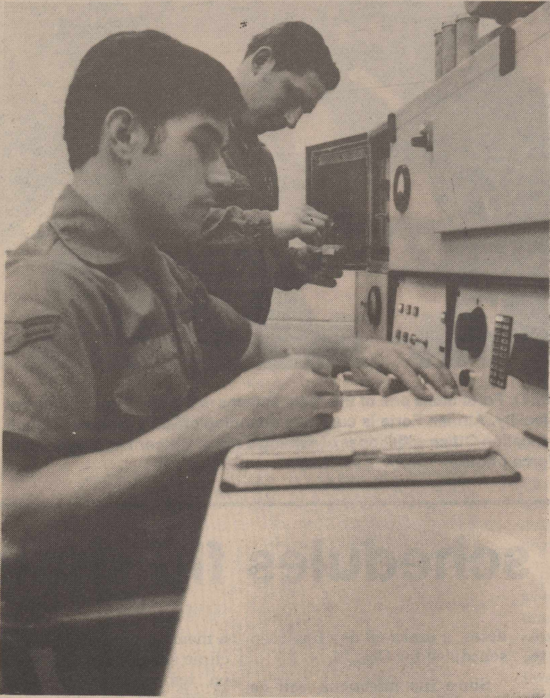
A1C Barry Cole and SSgt. Andrew Dollittle, above, run a test for foreign particles, such as metal shavings, in aircraft oil. The System Oil Analysis Program (SOAP) prevents damage by allowing NDI specialists to determine engine wear. A1C Denise P. Smith, below, checks a tech order while X-raying a part.
