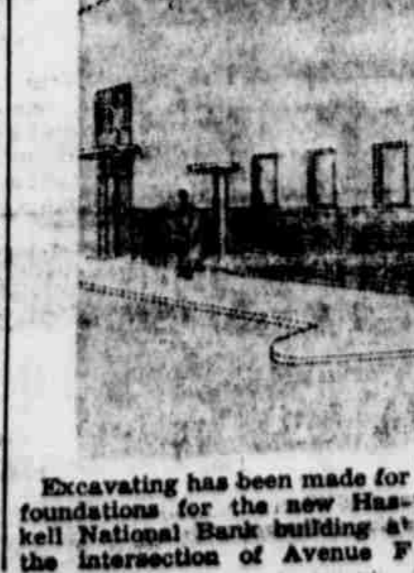
Excavating has been made for foundations for the new Haskell National Bank building at the intersection of Avenue F and North First Street.
