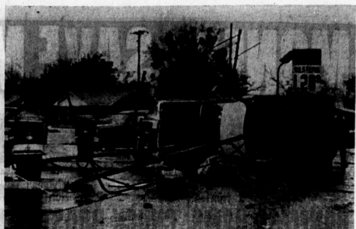
TWISTER'S PATH — A tornado slammed into the Bay Minette area near Mobile, Ala., Tuesday, destroying service stations, homes and the Bay Minette Middle School. Several students and a school bus driver were injured and numerous others suffered minor injuries. The school gymnasium was destroyed and several nearby homes were damaged. (AP Laserphoto)
