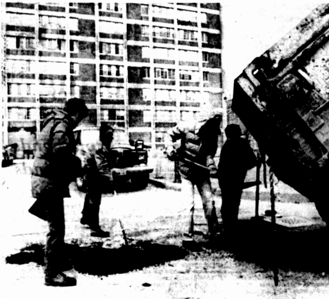
PAVING THE WAY — City workers fill in the potholes Tuesday in front of the building in the Cabrini-Green housing project where Chicago Mayor Jane Byrne and her husband, Jay
