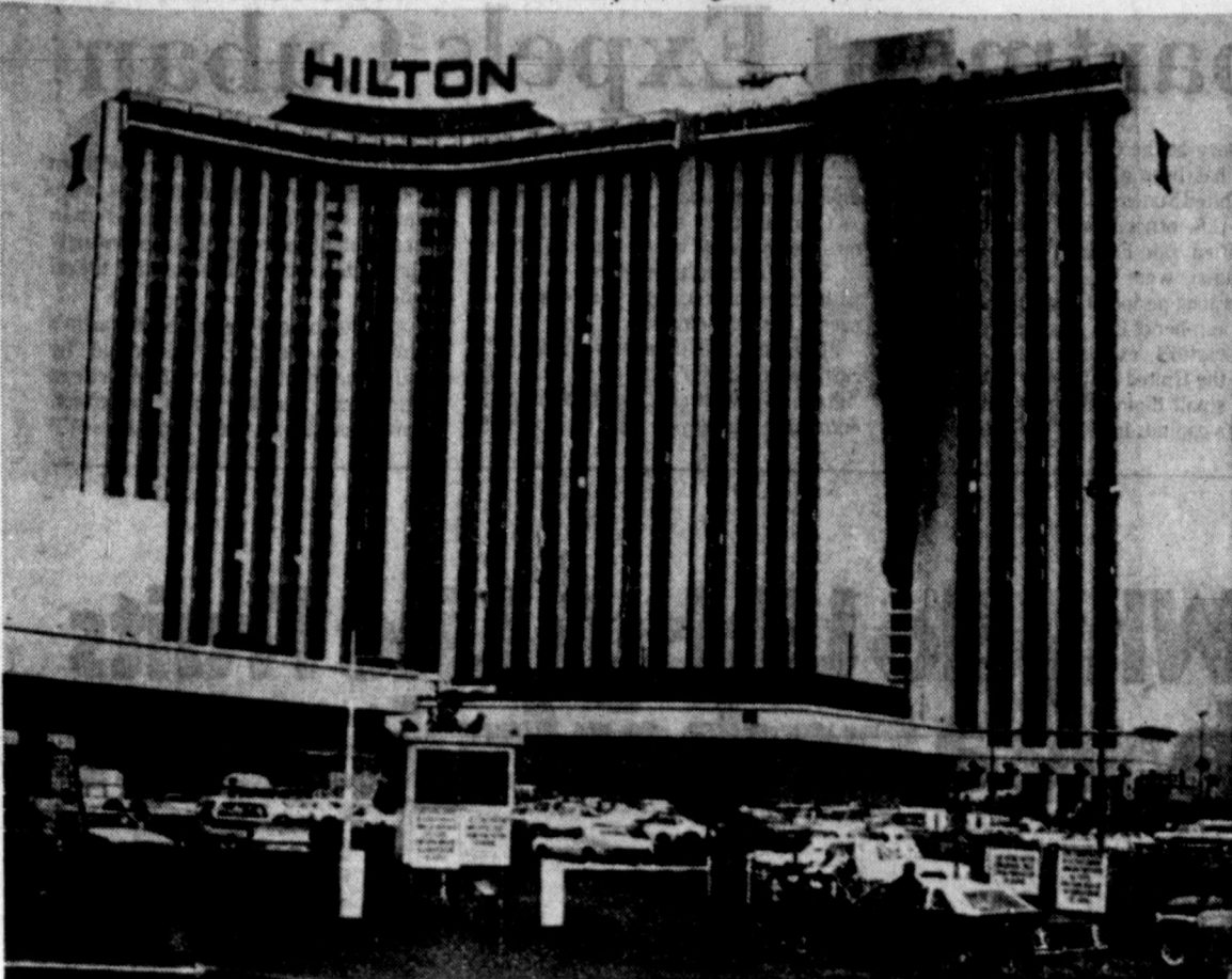
HOTEL BURNED — An exterior view of the Las Vegas Hilton Hotel shows the southeast wing charred from the eighth floor to the roof early Wednesday. Four fires of suspicious origin sent smoke throughout several floors of the 30-story hotel Tuesday night, killing eight people and injuring 242. (AP Laserphoto)
