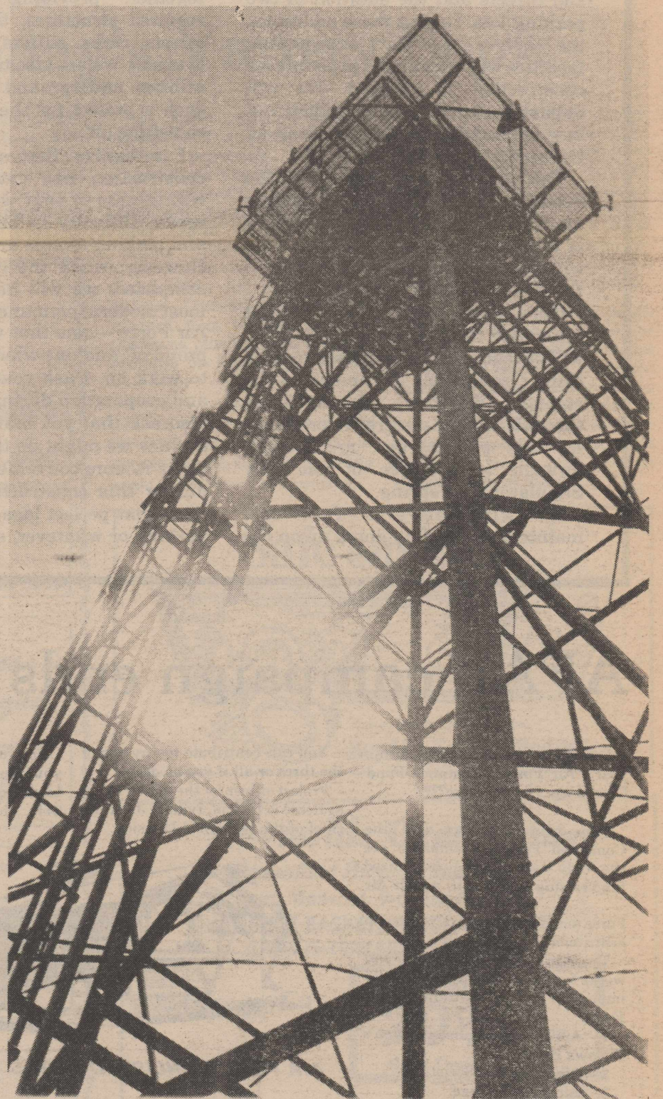
HIGH PLAINS SIFTER — FPS 77 weather radar sorts out a variety of information to assist Reese weathermen in making forecasts. The unit can track cloud targets within a 200-mile radius of the radar dome, and warn of approaching precipitation or severe weather. Reese and the National Weather Service Forecast Office, Lubbock, have agreed to an exchange of weather data. See story on page 4. (U.S. Air Force Photo by 2nd Lt. Mike Dale)
