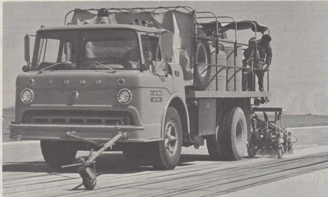
NEW STRIPES — A powerful striping machine sent in by Air Training Command paints almost instantly drying stripes on Reese runways. Here is the machine in action
