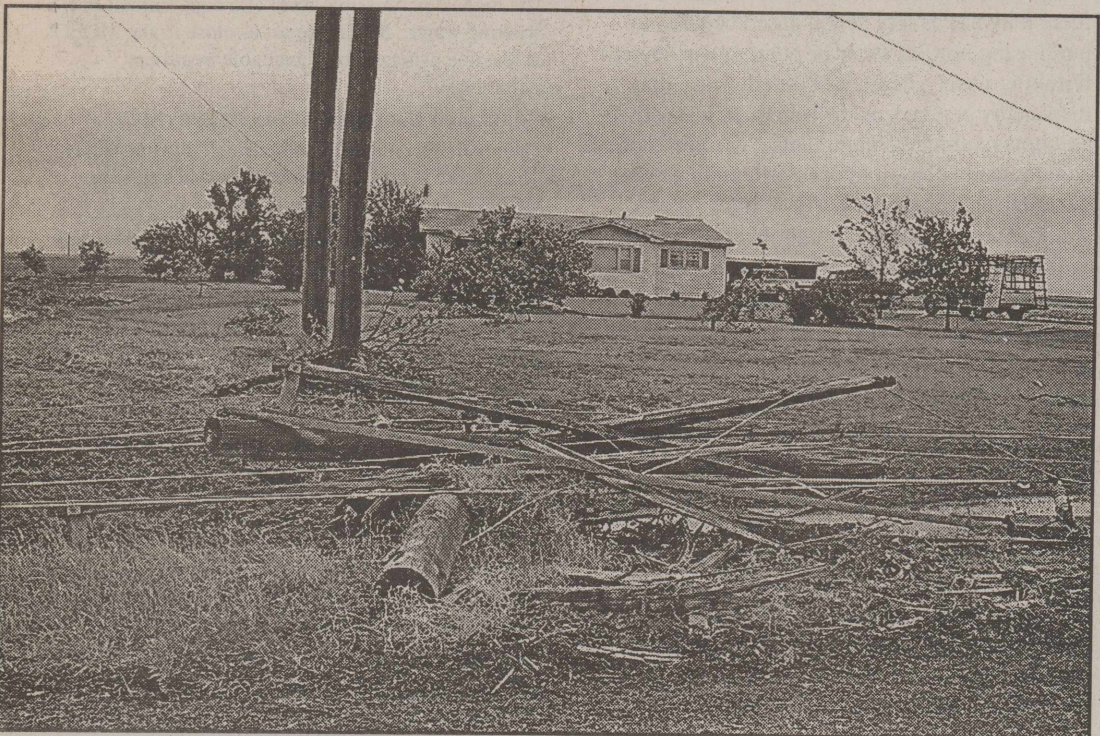
DOUBLE POLE STRUCTURES CRUMBLE IN THE ALLMON AREA--Double pole power line structures could not stand up to high tornadic winds in the Allmon Community. Remarkably the home in the background appears to have fared a little better than the poles. Staff Photo
