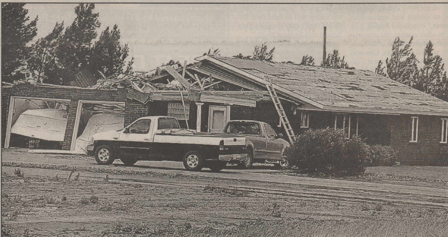
THE HOME OF MIKE KVETON, on Hwy. 54, between McCoy and Allmon, was heavily damaged by a tornado during the Thursday, June 9th, storm. The metal roof was completely torn from the house and the garage was destroyed. Debris from the home was dumped in an adjacent field. Mr. Kveton was at home during the storm taking shelter in a hallway. He was not injured.
