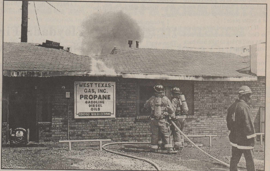
UNCLE'S (WEST TEXAS GAS) SERVICE STATION IN FLOYDADA WAS GUTTED BY FIRE--Wednesday, May 11, Uncle's, on north Hwy. 70, was gutted by a fire that started near an electric cook stove in the apartment side of the building, according to Fire Marshal Darrell Gooch. The gas pumps were not affected by the fire, nor the west storage building. West Texas Gas Operations Manager Cindy Lane said, "We plan to build a temporary building on location within a week to ten days to serve the public with fuel and the farmers with delivery of fuel. We are in the planning stages of rebuilding on site another convenience store. The old building has been declared a total loss." Staff Photo
