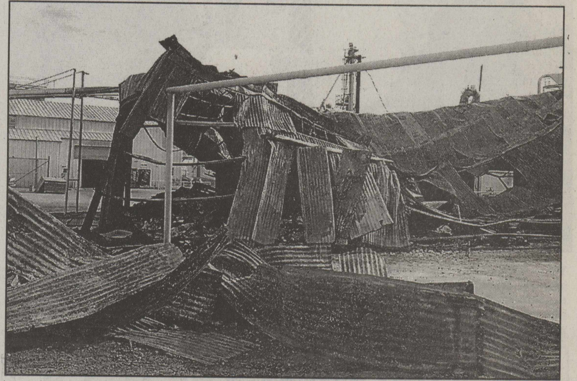
D&PL STORAGE BUILDING DESTROYED BY FIRE
