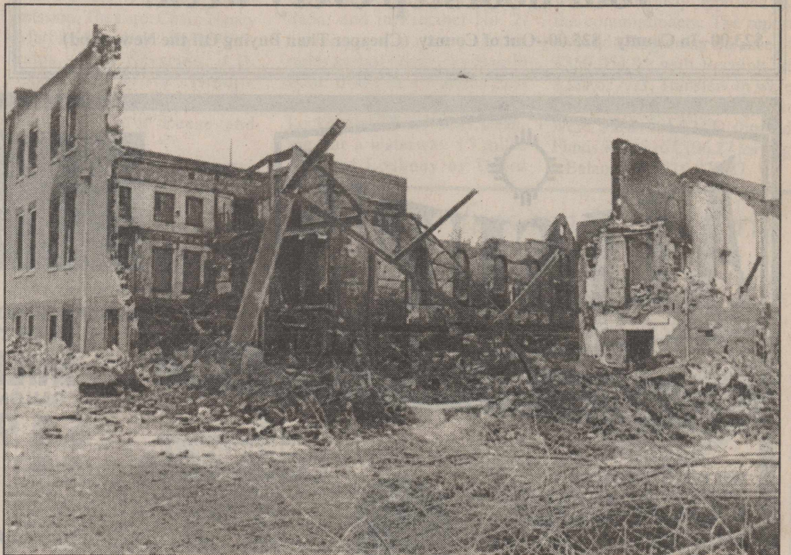
AFTERMATH OF FIRE ON THE MORNING OF MARCH 13, 2000
