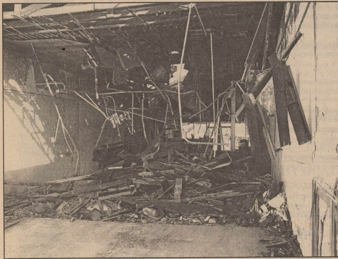
TEARING DOWN OLD DYSON'S BOOT SHOP —City crews were tearing out the old Dyson's Boot Shop on the west side of the square in downtown Floydada last Thursday. According to City Hall, the old building was causing water damage to the surrounding stores. Staff Photo
